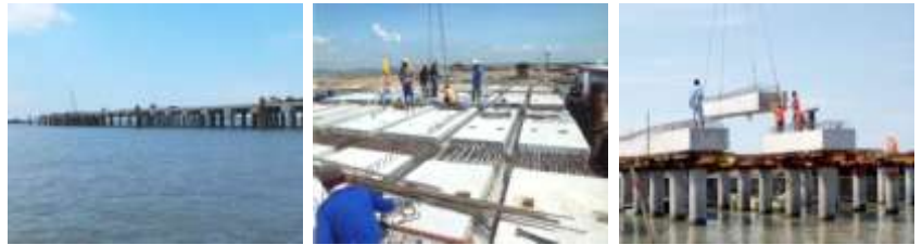
Trestle connecting the port and jetty is under construction.
