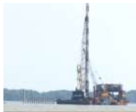
The piling work for jetty is ongoing.
