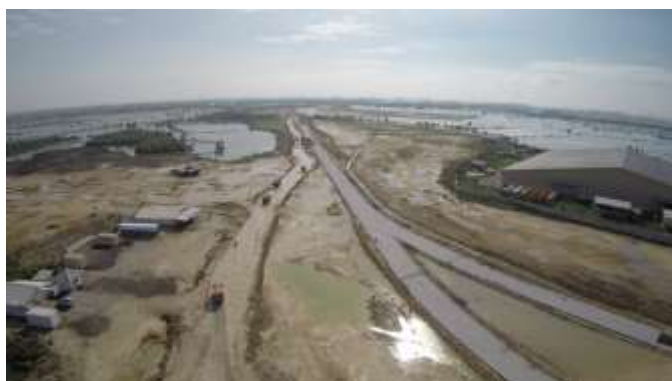
Industrial estate road infrastructure development
