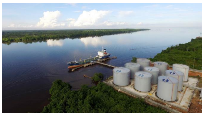
Pontianak Tank Terminal
