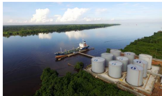
Pontianak Tank Terminal
