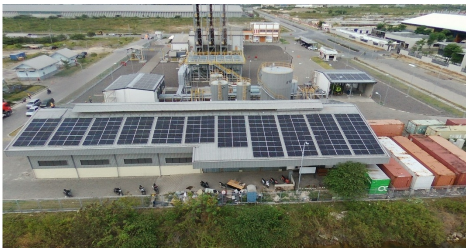
Rooftop Solar Panel JIPE
