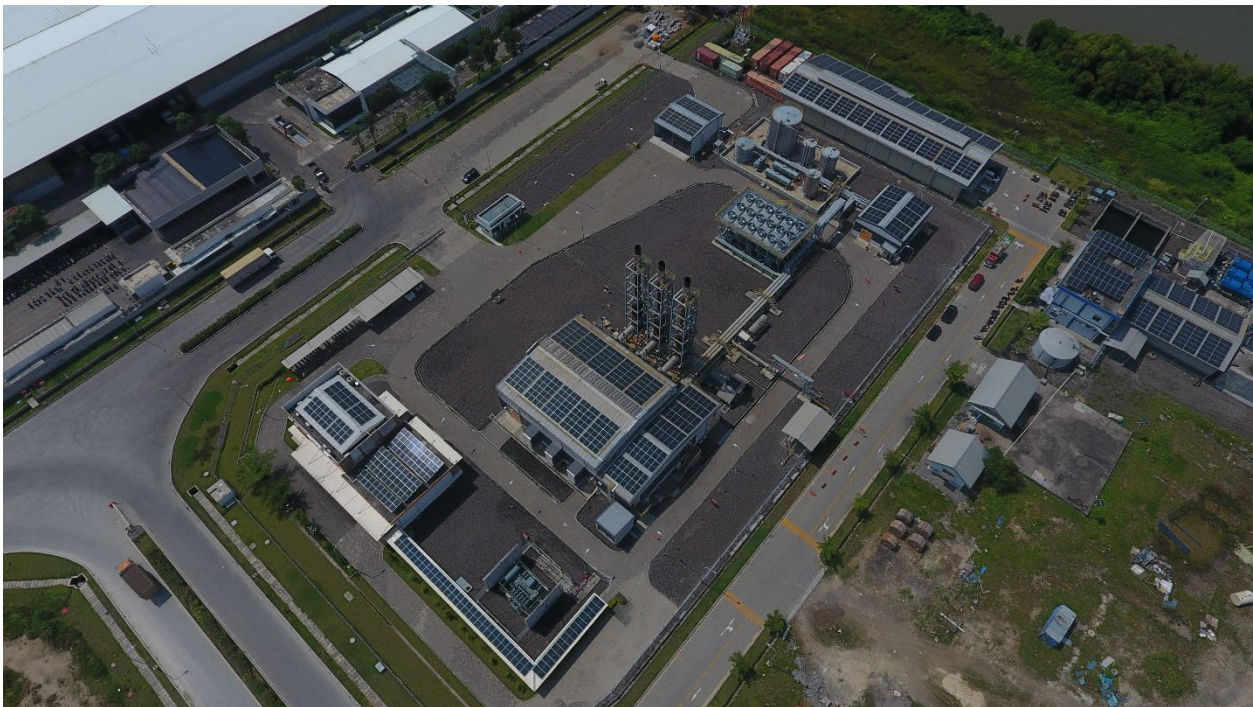
Solar Panel Installation in JIPE by XURYA
