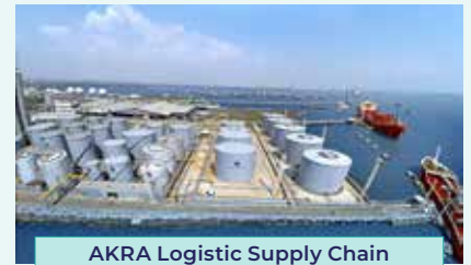
AKRA Logistic Supply Chain Infrastructure
