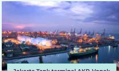
Jakarta Tank terminal AKR-Vopak
